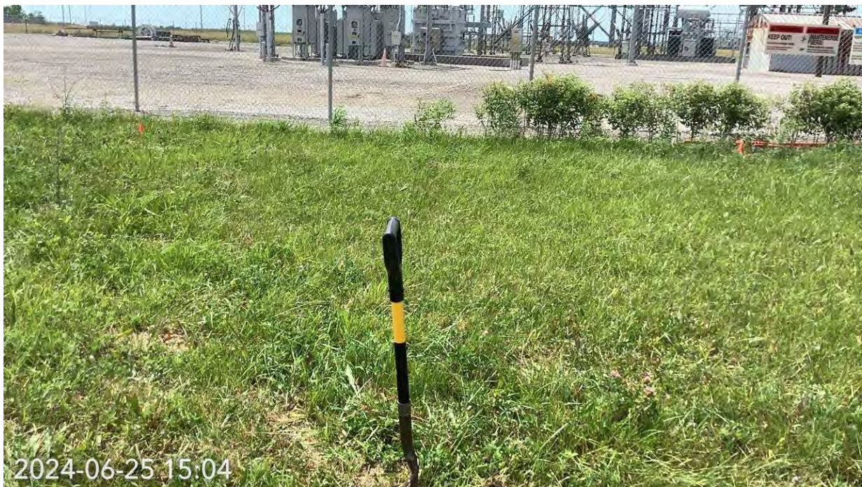
Photo Location 4. Representative view of maintained lawn and industrial land (existing Haviland Station) within the Project area. Photograph taken facing west.
